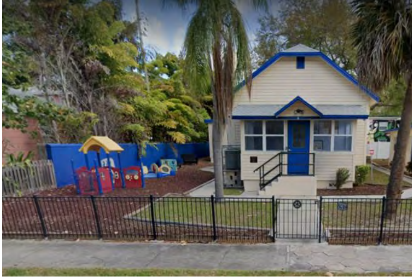
437 11 th Ave S. (Demolished)
