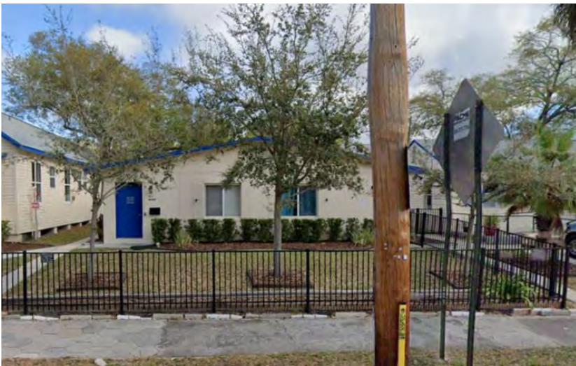
431 11 th Ave S. (Demolished)
