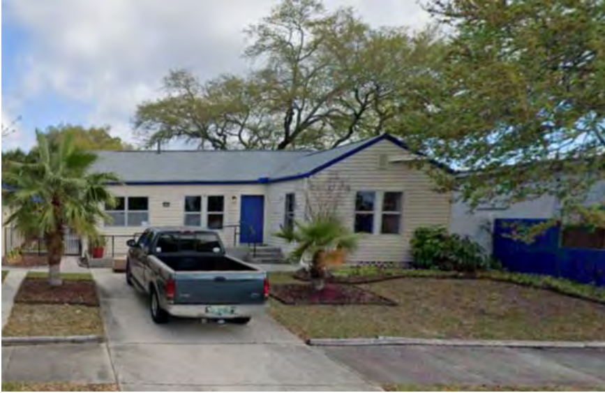
423 11 th Ave S. (Demolished)
